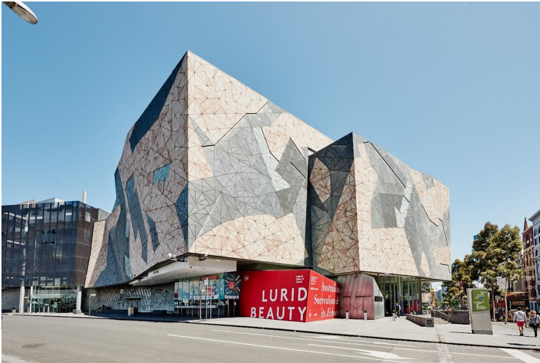
Ian Potter Centre (source: Hutchinson 2020)
